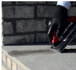
PIC 1. Fill joint with grout.
