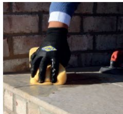
PIC 2. Remove excess grout with clean water.
